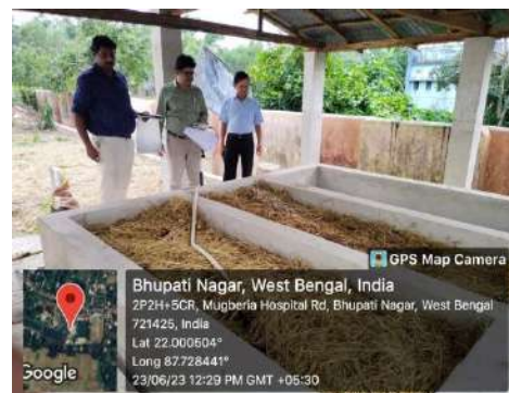
Organic waste Treatment unit ( Vermi Compost)
